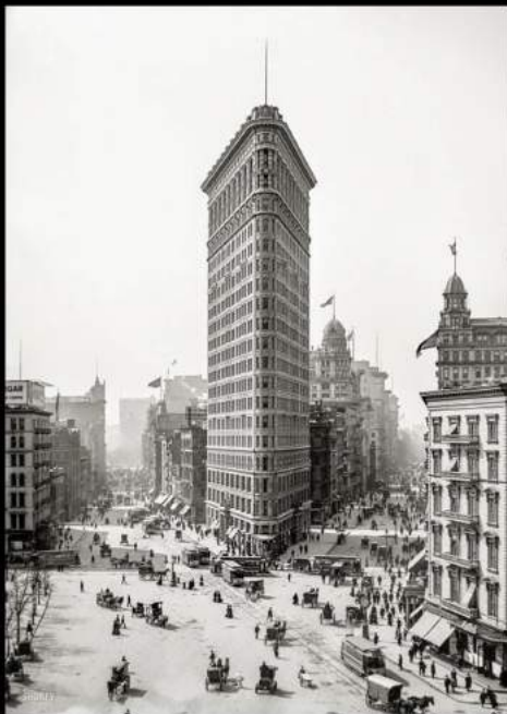
Daniel Burnham Flatiron Building
